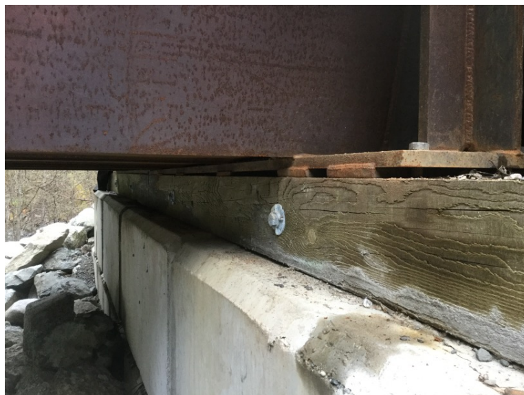
Steel shims downstream left bank
