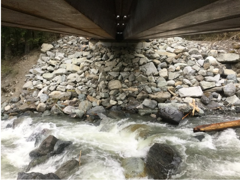
Right Bank Abutment when facing downstream
