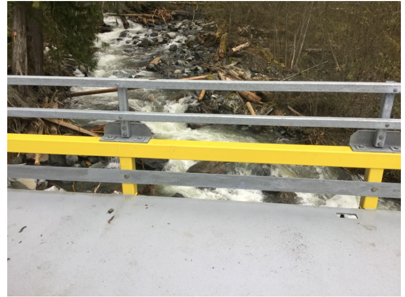
Handrail and footrail
