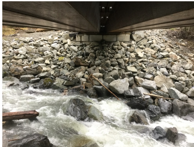
Left Bank Abutment when facing downstream
